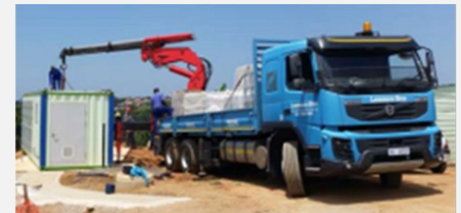
Figure 16: Installation of a sanitation management system in South Africa. © Woodco Energy
